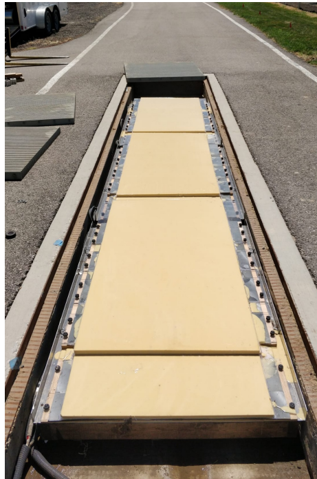
Fig. 5.16: Three primary pads potted and placed in the outdoor trench.
