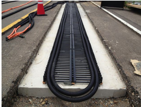
Fig. 1.7: Elongated rectangular track coil used for wireless charging [9].
