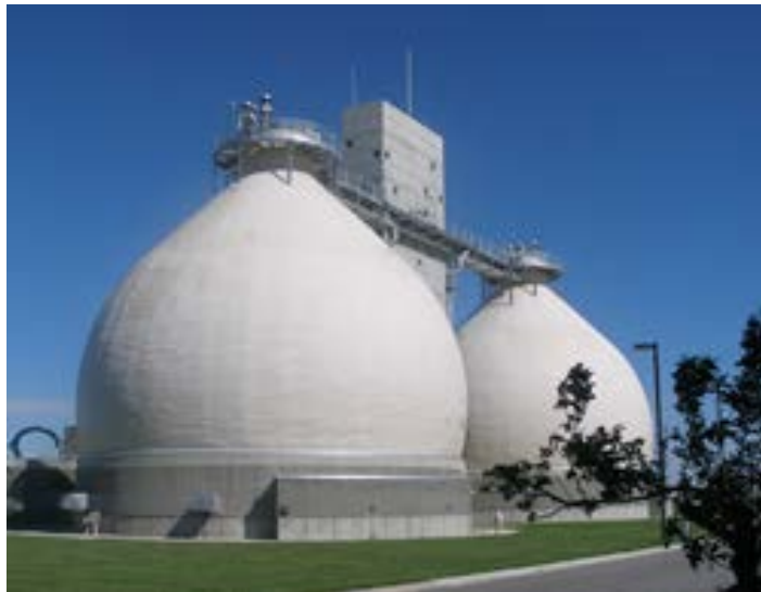
Central Valley Water Reclamation Facility Anaerobic Digesters
