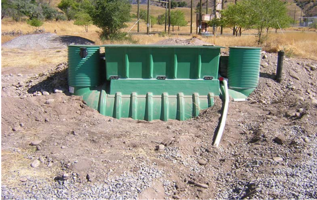
Installation of alternative on-site systems for different soil types.
