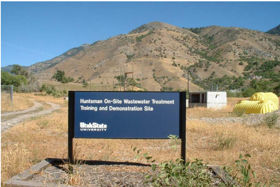
The Huntsman On-Site Wastewater Treatment Training and Demonstration Site
